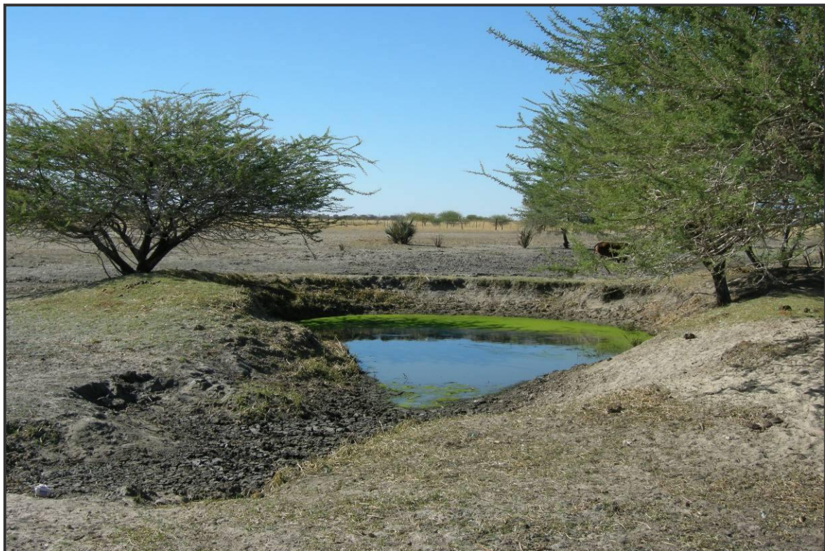
Figure 11: Shallow hand dug well ( omithima ), not fenced off and therefore used for livestock watering
