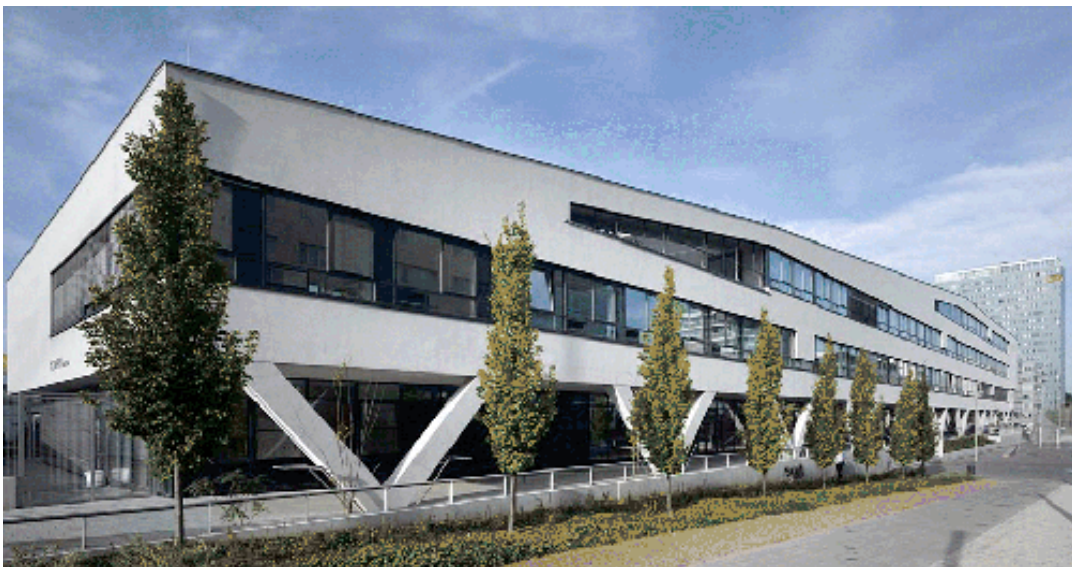
Abb. 20: Campus Monte Laa (URL: http://www.nmpb-architekten.at/index.php?section=51&id=8&id_gal=46&id_gal_sel=581 ; Zugriff am 24.08.2010)
