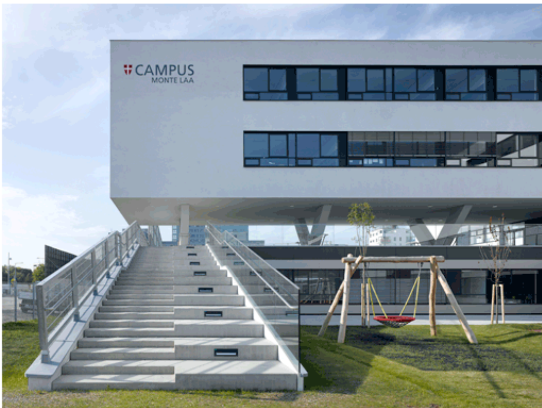
Abb. 16: Campus Monte Laa (URL: http://www.nmpb-architekten.at/index.php?section=51&id=8&id_gal=46&id_gal_sel=551 ; Zugriff am 24.08.2010)
