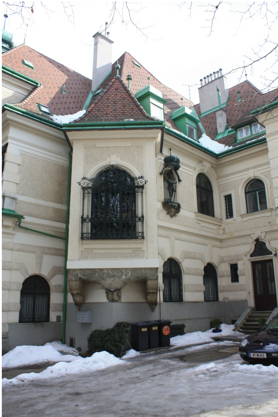
Abb.31: Fassade Villa Schoeller / Winter 2009
