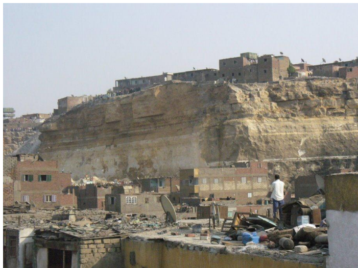
Figure 14 Al-Duwaiqa after the rock fall (Picassa 2008).
